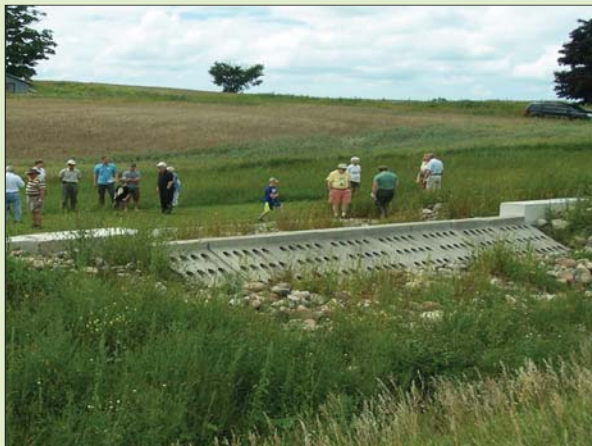
Appreciation Day bus tour takes local residents on a tour of recent projects. Seen here is the Eadie Berm, designed to slow down water and reduce soil erosion. Funding for this berm was provided by Environment Canada, County of Bruce and the Ontario Ministry of the Environment and Climate Change.
