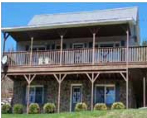
highlights porch with post, side brace and exposed beams
