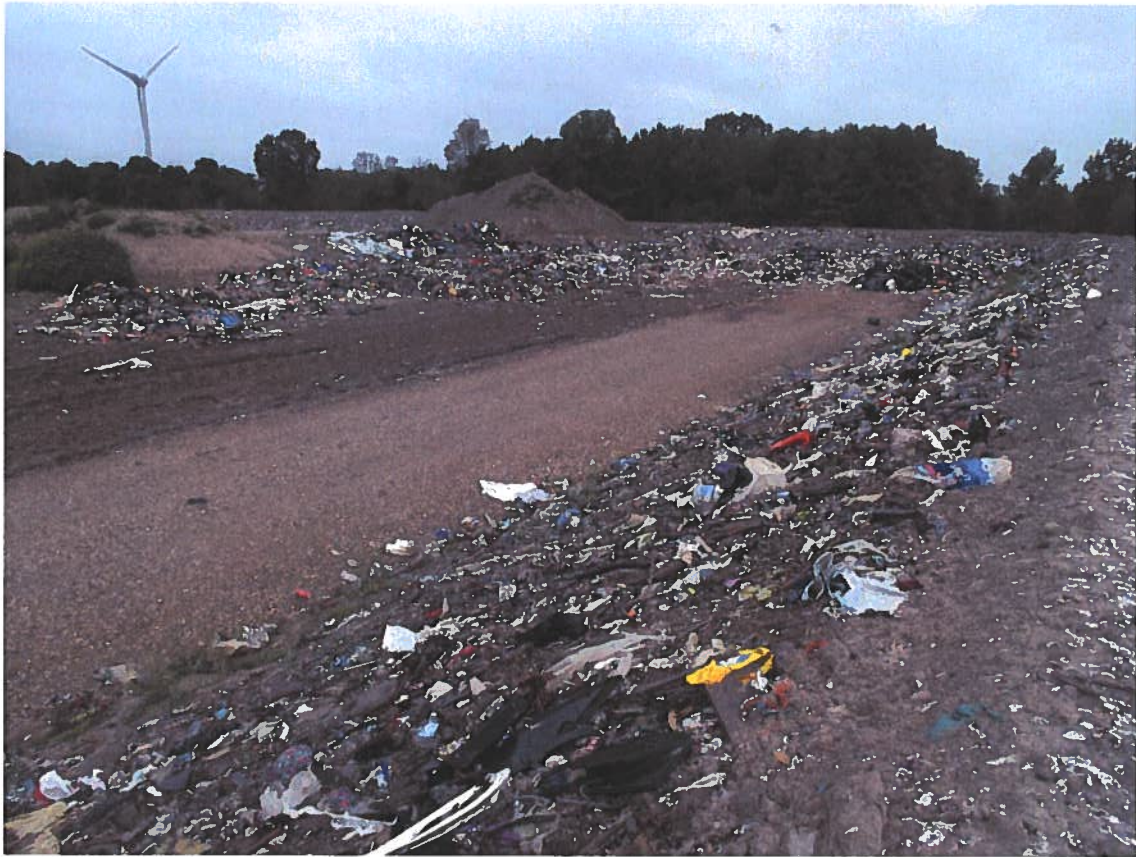
Photo showing exposed waste along active area access road and large active face of landfill.
