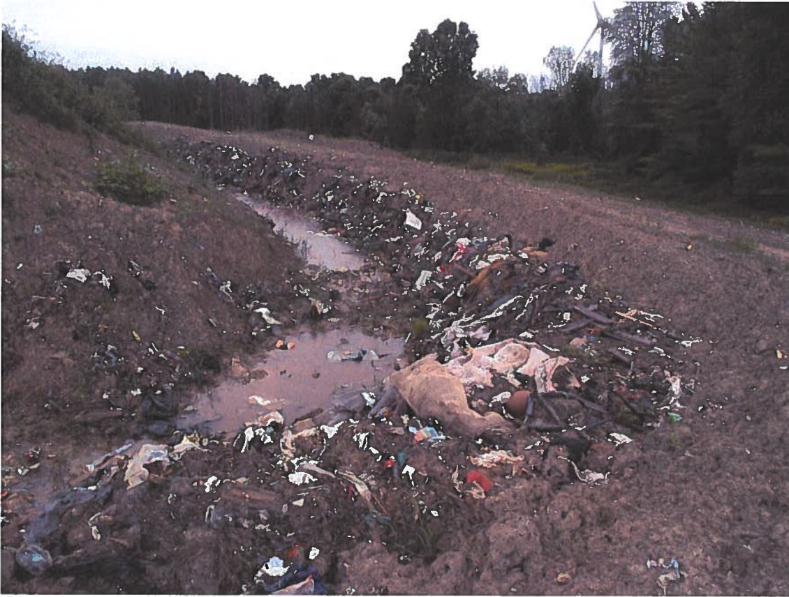
Photo showing ponded water and leachate in waste .
