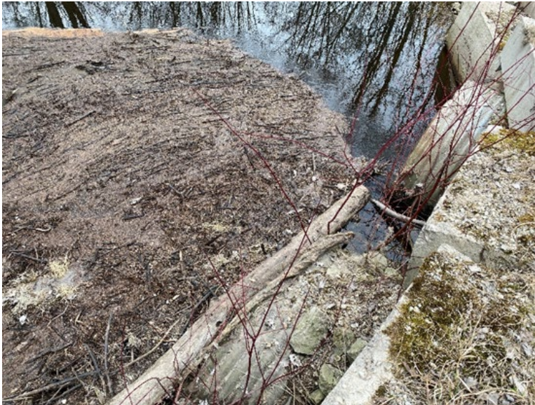
Figure 7: Upstream End of Culvert with Blockages (Sta. 2+558, Facing West, April 11, 2023)
